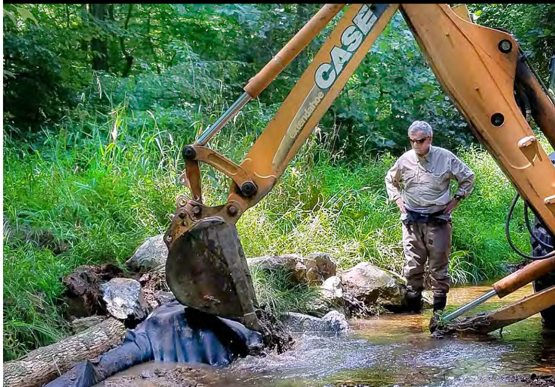
Stream restoration: Jay Lovering at the Conewago workday.
